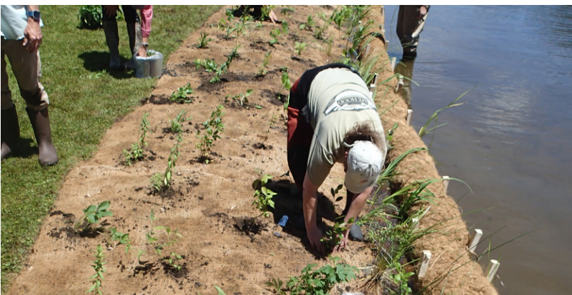
Bioengineering project being installed as part of the Michigan Natural Shoreline Partnership Certified Natural Shoreline Professional (CNSP) Training
